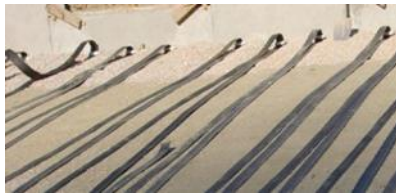
(a) Placing polymer strip reinforcements
