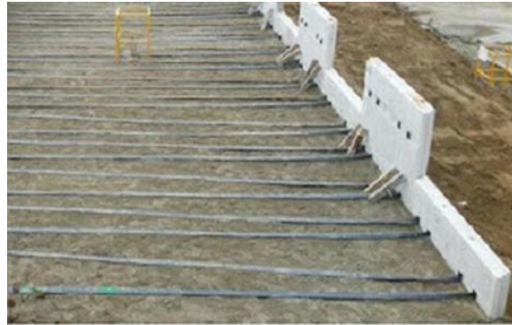
(c) General overview of wall and prefabricated front face elements
